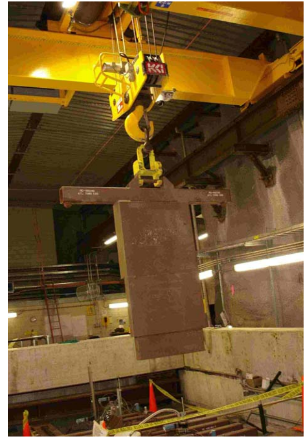
Steel shielding block being moved.
